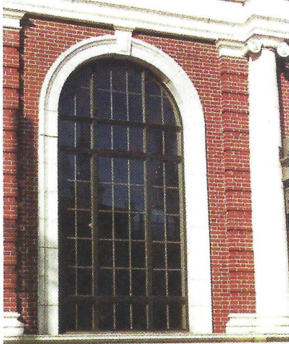
Custom-designed storm windows are available for very large openings, as seen here at Covington Station in Covington, KY.
